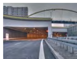
Stadstunnel in Polen 72
