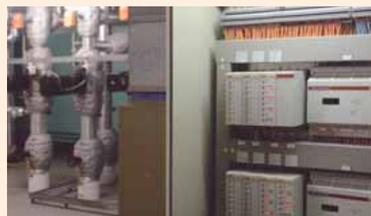
▲ Primary facility at the AMC hospital with «veteran» Saia®PCD4 and Saia®PCD2 in the control panel.
