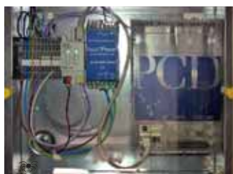
◀ Saia® PCD1.M2120 EIB/web connection to the existing EIB network
