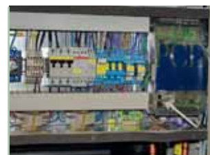
▲ View of ventilation tower control panel with Saia®PCD1
