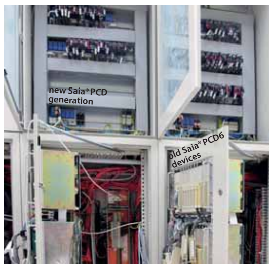
▲ Pictures of the new (top) and old (bottom) panel: The new panel was fitted with Saia PCD 3 and tested without stopping production using the "old" Saia®PCD6 devices.
