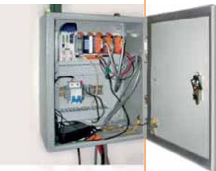
▲ PCD3 to record meter values – everything is not always installed entirely in line with standards
