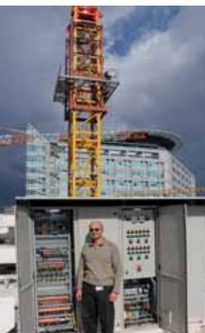
▲ The control panel is located on the roof of the hospital under the fierce sun rays of the Middle East: that posed a challenge for the PLC technology!
