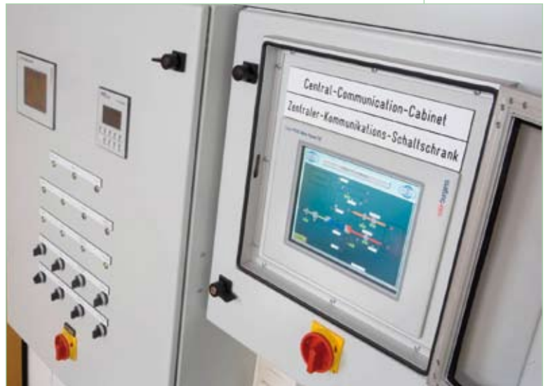
Central communications cabinet at HANSA's headquarters: Web access to every application in the field.
