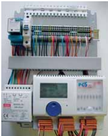
Its common heating system is controlled by a Saia®PCD3.M5540 gateway station. This has 6 interfaces in multi-pro-
