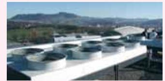
Coolers on hotel roof
