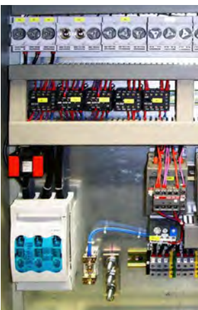
▲ Stroomtrafo in schakelkast
