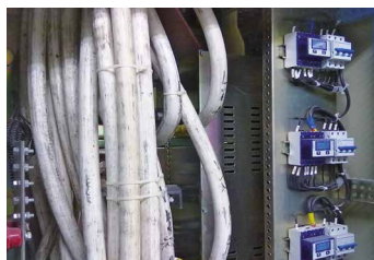
▲ Energy meters in tough industrial environment
