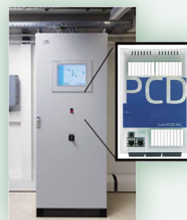
Potential use in primary switch cabinet
